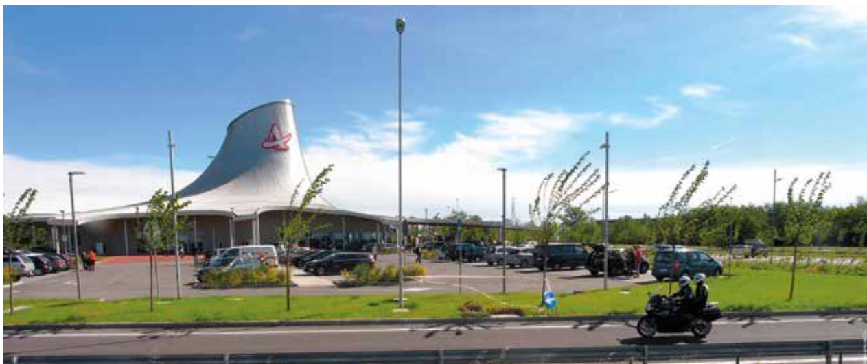
Autogrill Villorese EST, primo Ecogrill certificato LEED / Autogrill Villorese EST, first LEED certified service station
