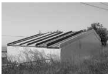
Caso studio A (coperture LV6-A, LV6-L, MV6-A, MV6-L, LV3-A)
